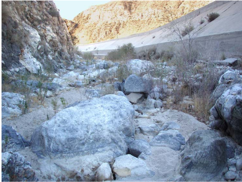
Figure 3-20. Relatively rapid delivery of anorthosite (crystalline) rock boulders into the USCR from steep, nominally shrub-covered hillslopes along Soledad Canyon. Note the presence of the Southern Pacific Railway on river right, which further constricts the canyon reaches of the USCR.
