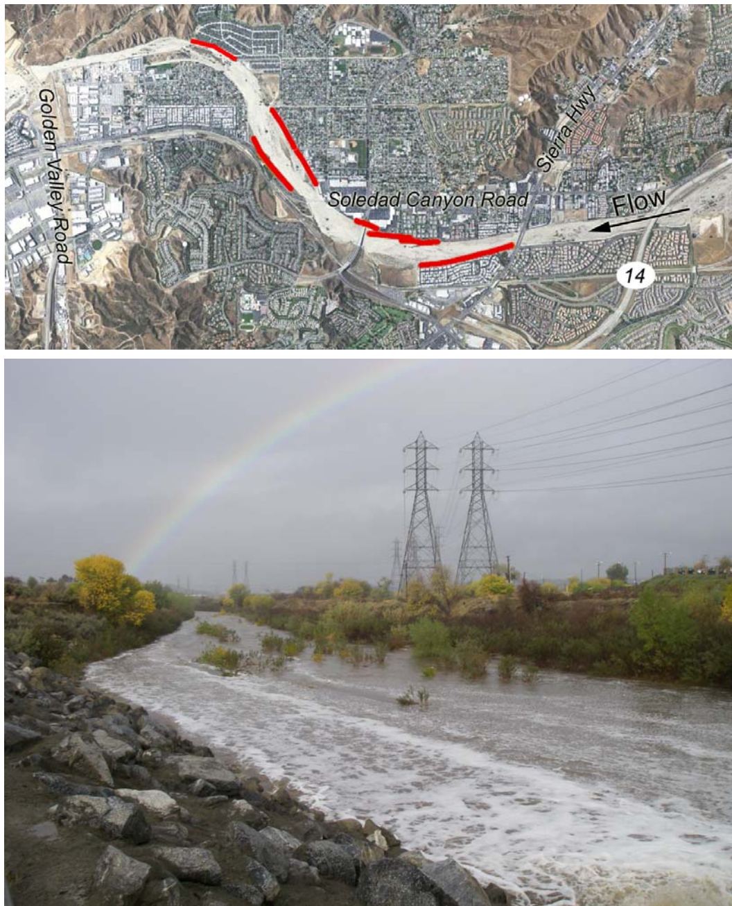
Figure 4-11. Floodplain developments and flood control structures (non-federal levees shown in red [source: CDWR 2009]) in the Santa Clarita basin. Dense urban developments on the floodplain, adjacent to the river channel, and roads crossing the river are shown in the NAIP 2009 aerial photograph (upper) of the eastern end of Santa Clarita near the Mint Canyon confluence (right side). Hardened banks with rock revetment on the left bank and an earthen levee along the right bank of the downstream end of the South Fork SCR are visible in this photo (lower) taken during high flows on 12 December 2009.
